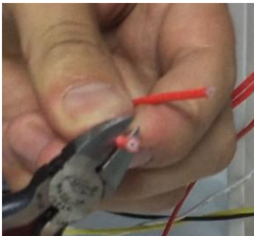
Use the tool to strip off the cord.
